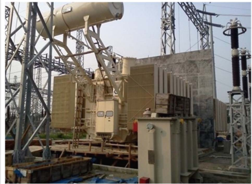
Fabrication of 230kV Transformer(Nov.09, 2012)
